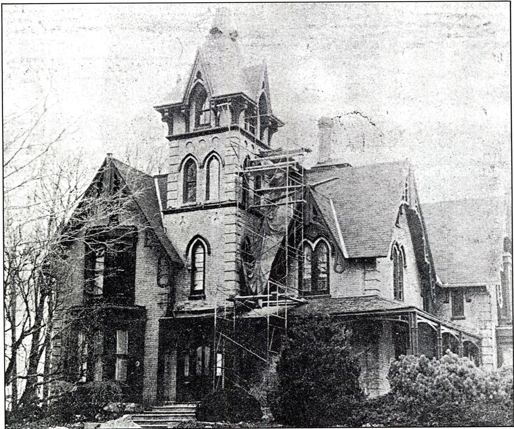
ELMHURST IN THE 1970's, UNDERGOING RENOVATION AS A RESTAURANT.
